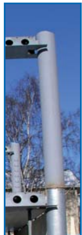
Figure 9. Deltabeam with round column
