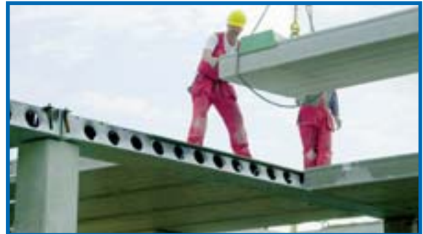
Figure 11. Position of the end of a hollow-core slab in relation to Deltabeam
